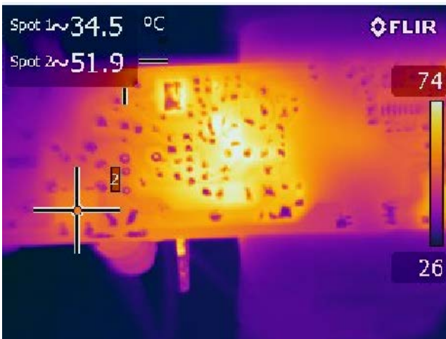
Figure 35 – 230 V VAC, Full Load. Spot 2: Bridge Diode (BR1): 51.9 °C.
