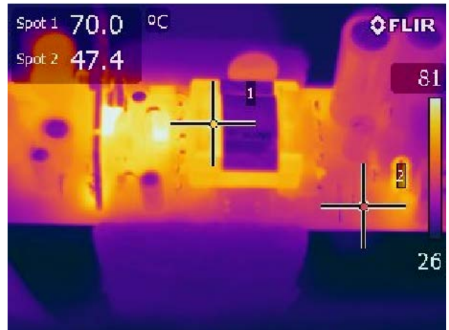
Figure 38 – 170 V VAC, Full Load. Spot 1: Transformer (T1): 70 °C.
