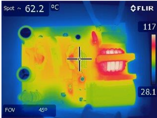
Figure 18 – Transformer Side. 115 VAC, Full Load.
